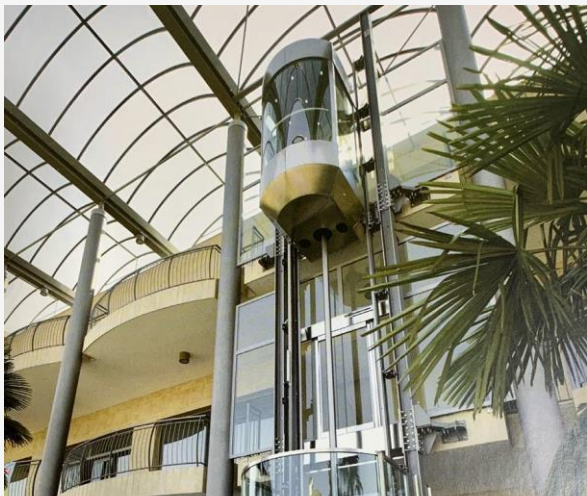
Supporting structure for lift
